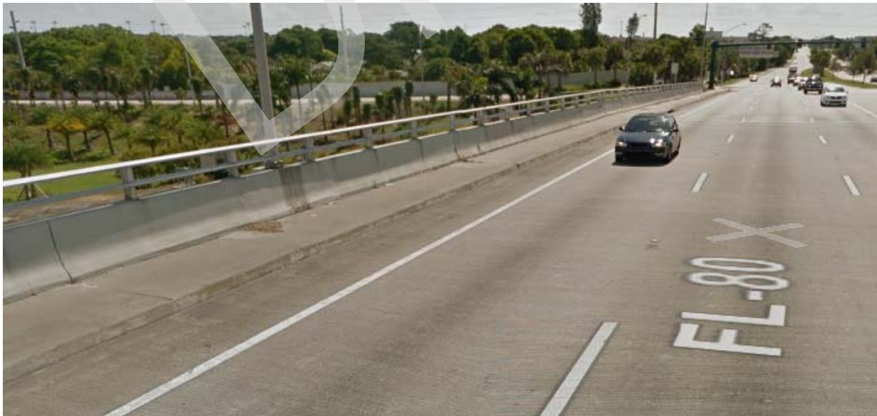
Figure 3.5: SR 80, Sidewalk and Bicycle Lane over I-95
